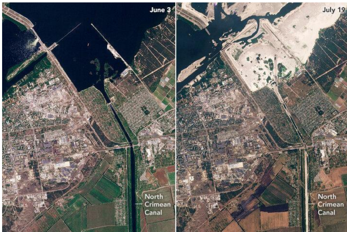
The location of the North Crimean Canal water intake from the upstream side of the Kakhovka HPP Dam (southern part of the Kakhovka Dam) before and after the dam was blown up. Source: earthobservatory.nasa.gov
