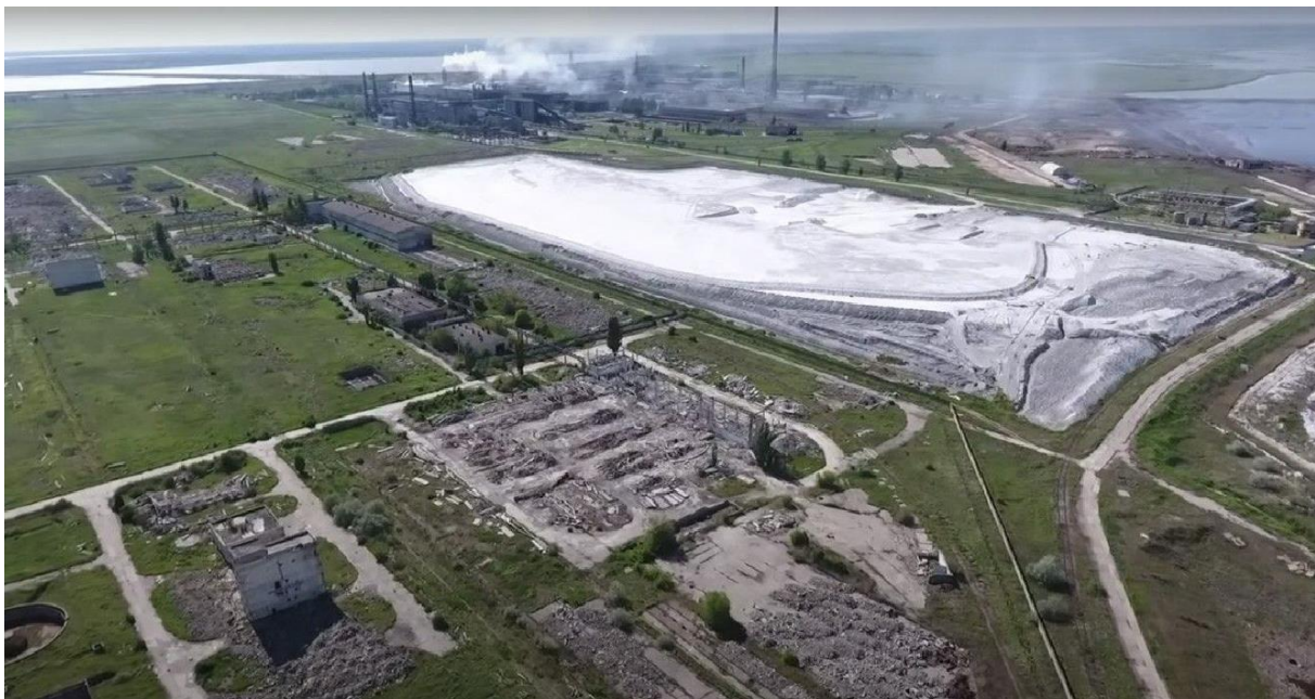
View of the acid accumulator of the Crimean Titan Plant, 2018 152
