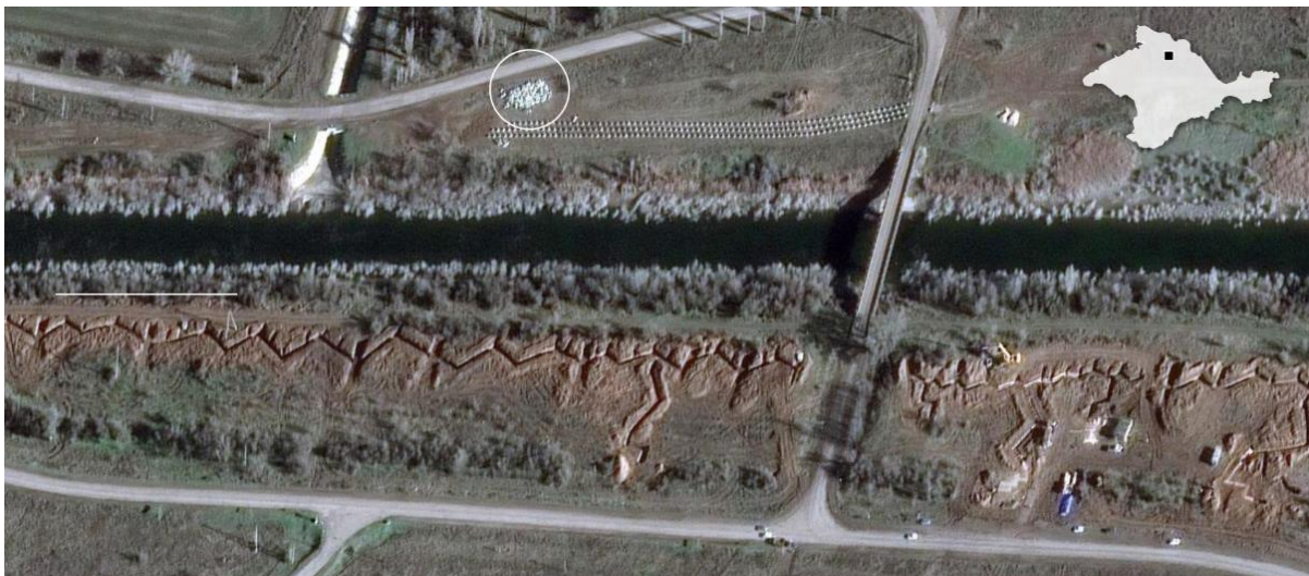
Trenches and “dragon’s teeth” along the banks of the North Crimea Canal. Source: https://www.washingtonpost.com/world/interactive/2023/ukraine-russia-crimea-battle-trenches/?itid=hp-top-table-main_p001_f001
