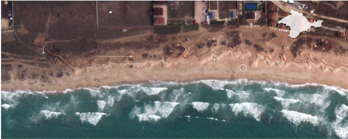
Section of Russian engineering fortifications near the village of Vitine (12 March 2023). The photo shows trenches and even “dragon’s teeth” along the coastline. Source: https://www.washingtonpost.com/world/interactive/2023/ukraine-russia-crimea-battle-trenches/?itid=hp-top-table-main_p001_f001
