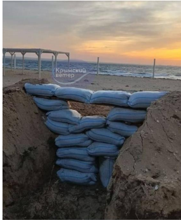
Engineering fortifications in Mizhvodne, 18.12.2022 https://t.me/Crimeanwind/18323
